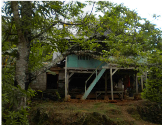
My house in Labundo. It was built on stilts to keep the snakes out.
