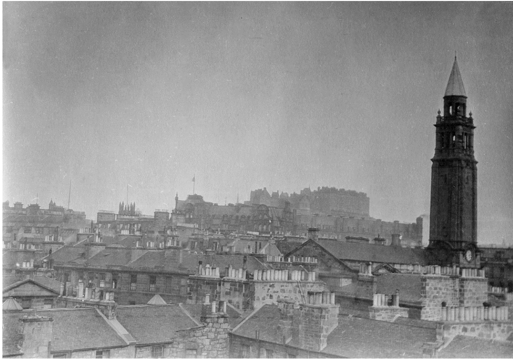
From the roof of 38 Melville Street, June 1931
