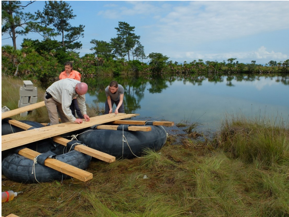
Figure 3: Constructing the coring platform
